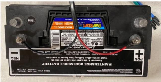
Battery with cable attached to terminals
