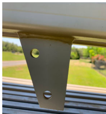
Predrilled holes for attaching electronic latch.
